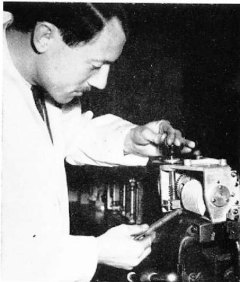
Arthur Partridge, Machine Shop, adjusts the condenser unit of a TF 370F Universal Wavemeter
